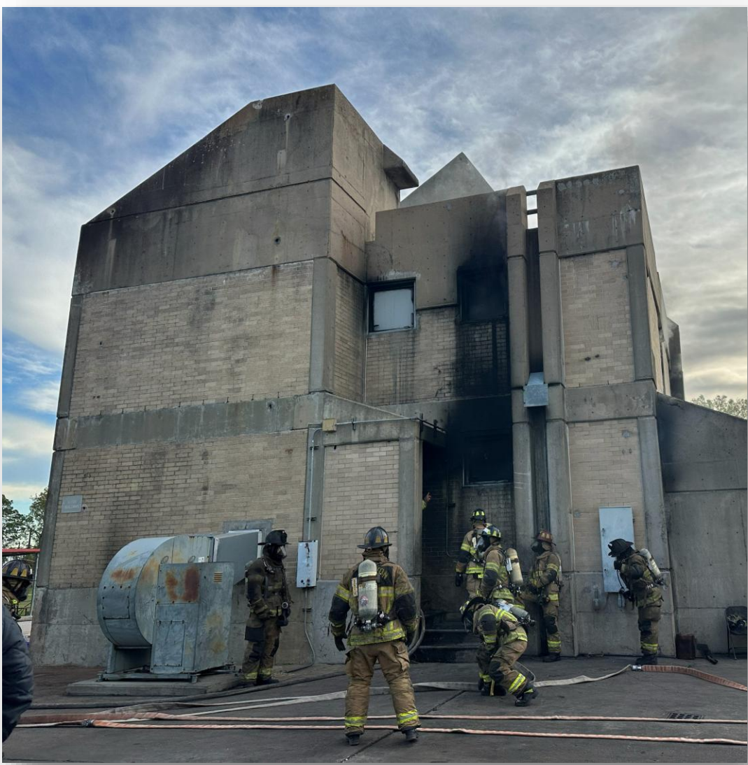
Figure 1. Two-Story Concrete Live-Fire Building.
